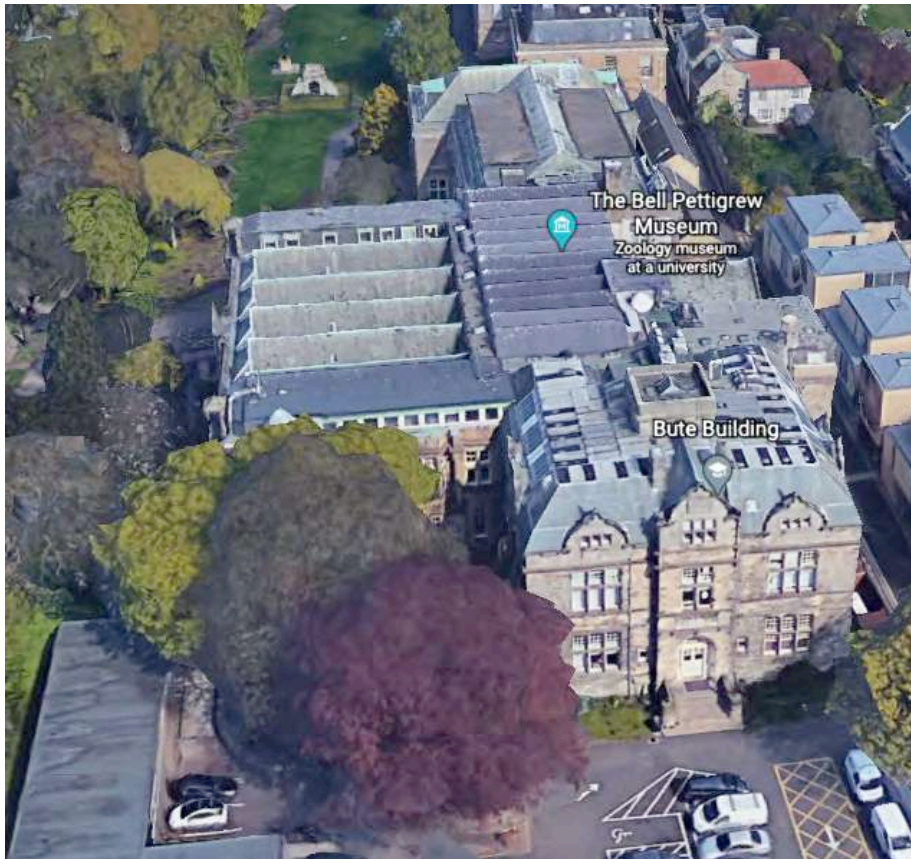
Bute Building from the air (Google Earth), home to SEES next year.
