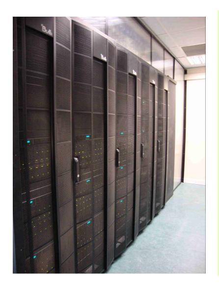
110 x 32-core compute nodes 128GB – 1.5TB memory each 2 nodes have GPUs (Tesla V100) 400 TB disk space
