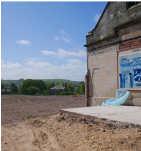
'New College' – with the demolition work complete.
